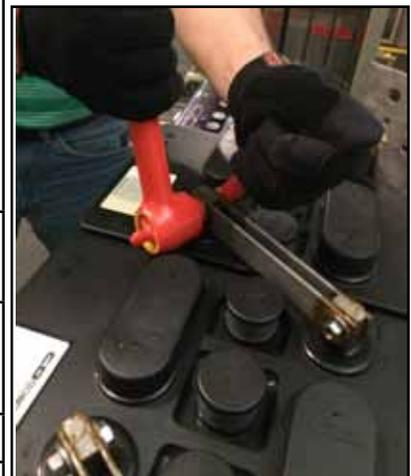
**FIGURE 1.4.7 - Torquing connections**
